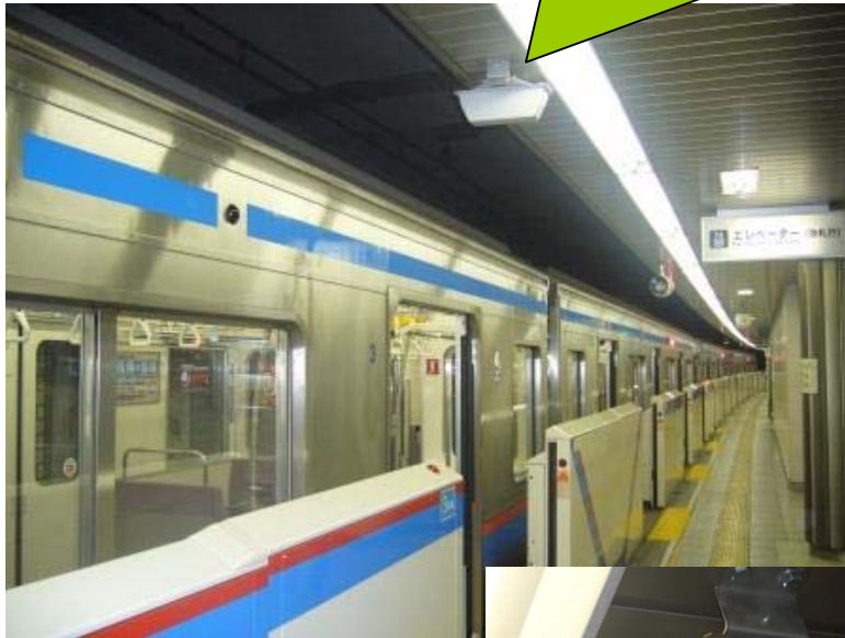
Antenna for re-transmitter mounted on ceiling of station
