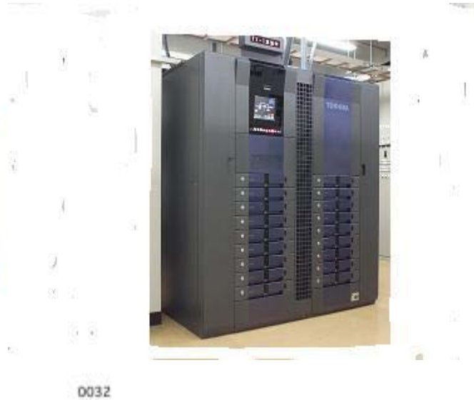
3 kW digital transmitter rack
