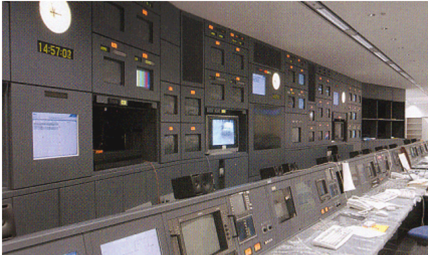
Master Control Room
